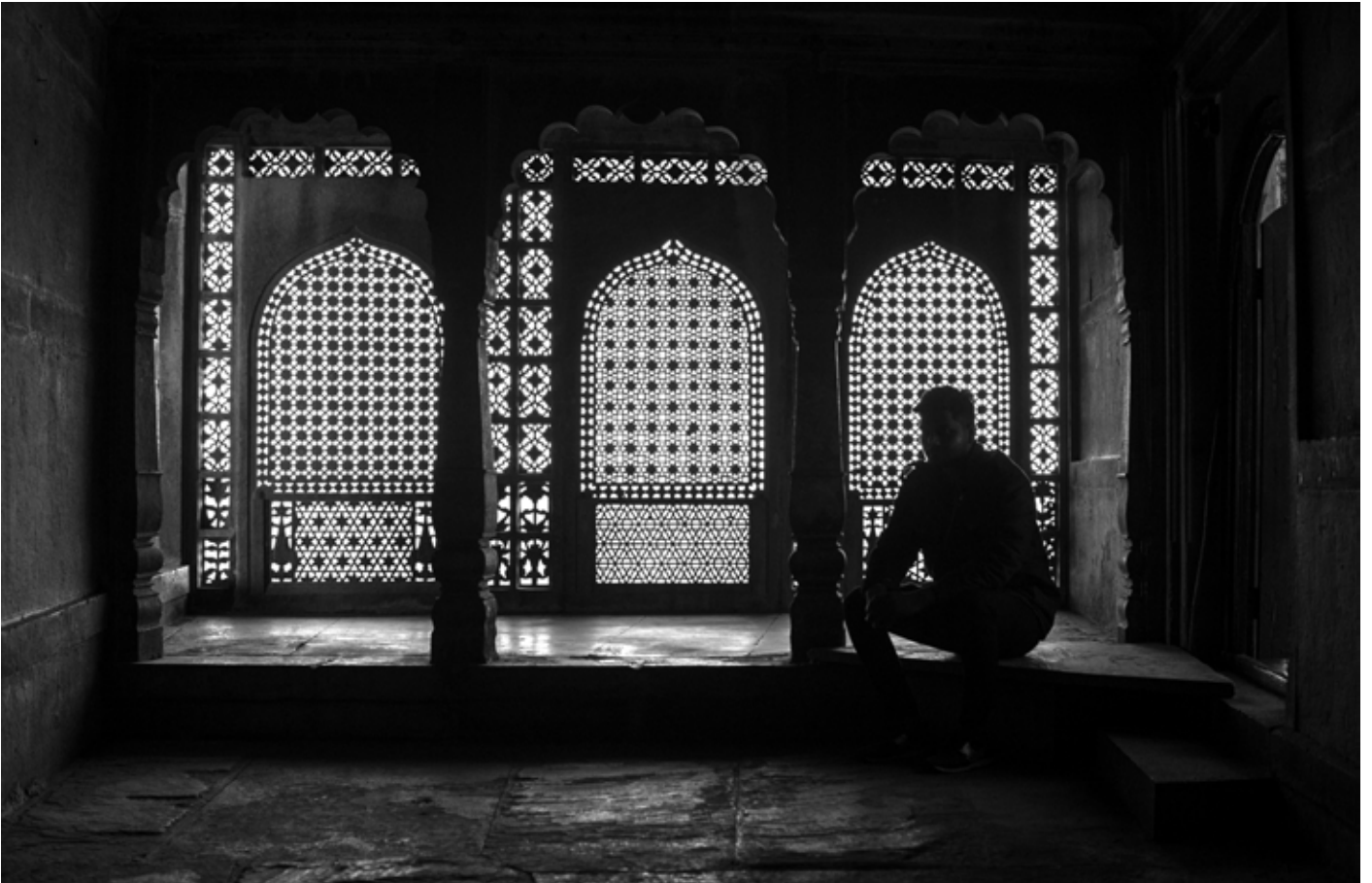
Intricate Jali Work on the south - west facade of the palace to have diffused light in the circulation spaces.
