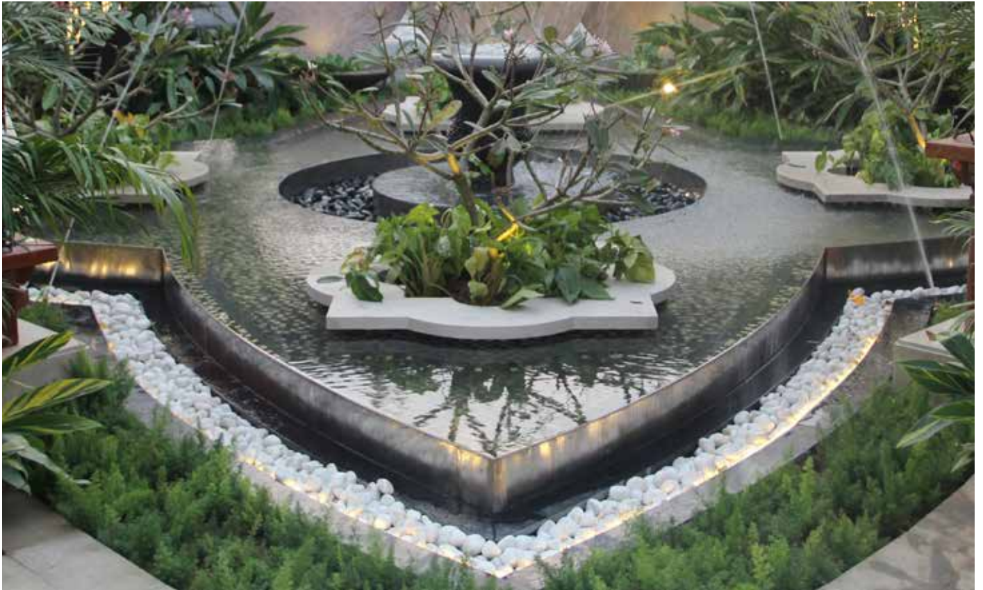
Top: Locally available stones innovatively used in gabion wall structure and flooring pattern. Bottom: Use of metal edging to achieve the traditional lotus petal shaped edge for the water feature.
