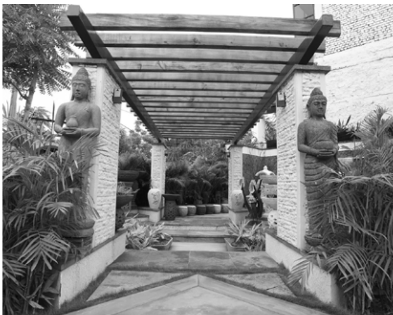
Cast in situ butch stones work on the pillars, with wooden trellis
