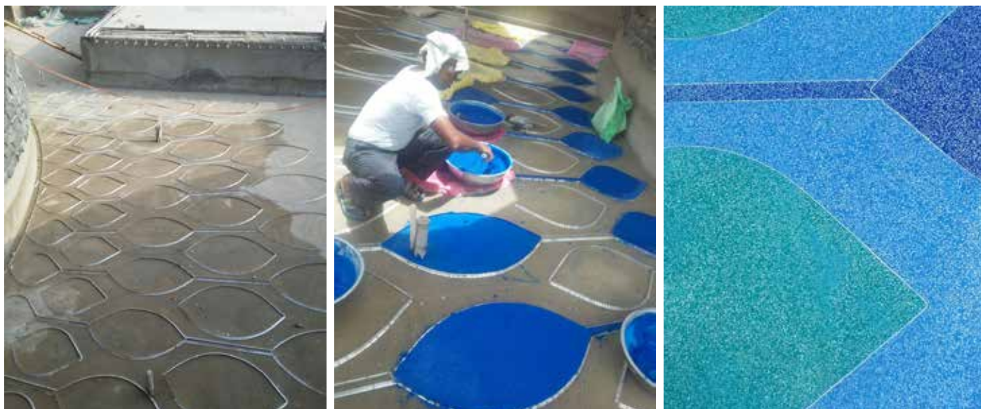
Cast in situ terrazzo in the water feature, using an innovative blend of colours and aggregates
