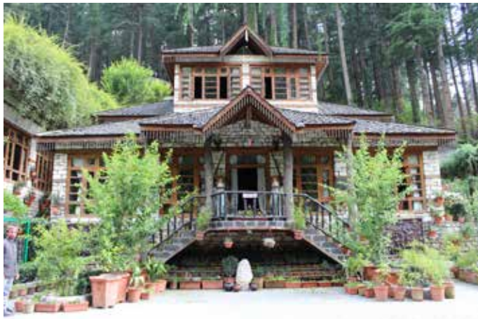
Figure 5: Reception block with raised plinth level with respect to natural topography
