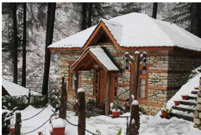
Figure 7: Snow-covered slate roofing
